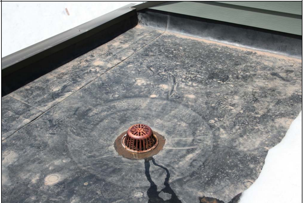
Notes: Roof Photo #1.
