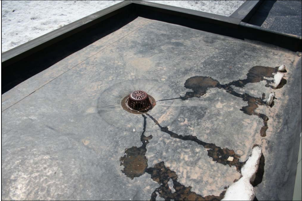
Notes: Roof Photo #2.
