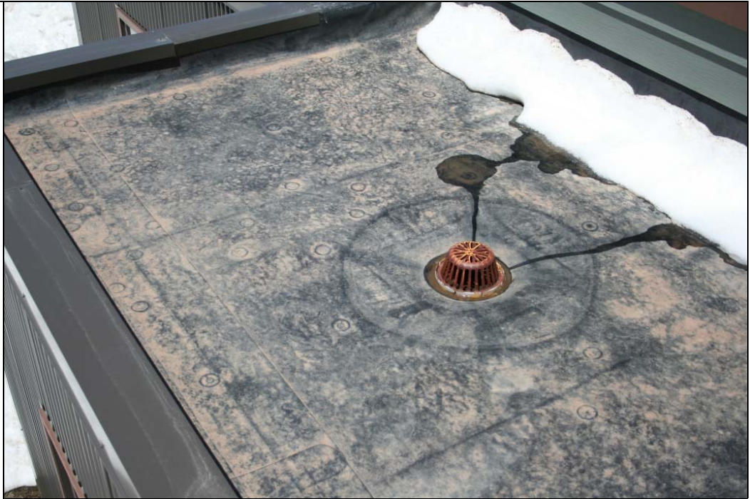
Notes: Roof Photo #1.
