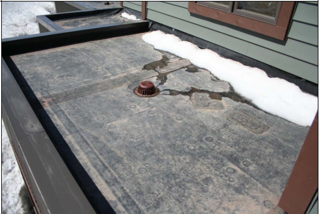
Notes: Roof Photo #1.
