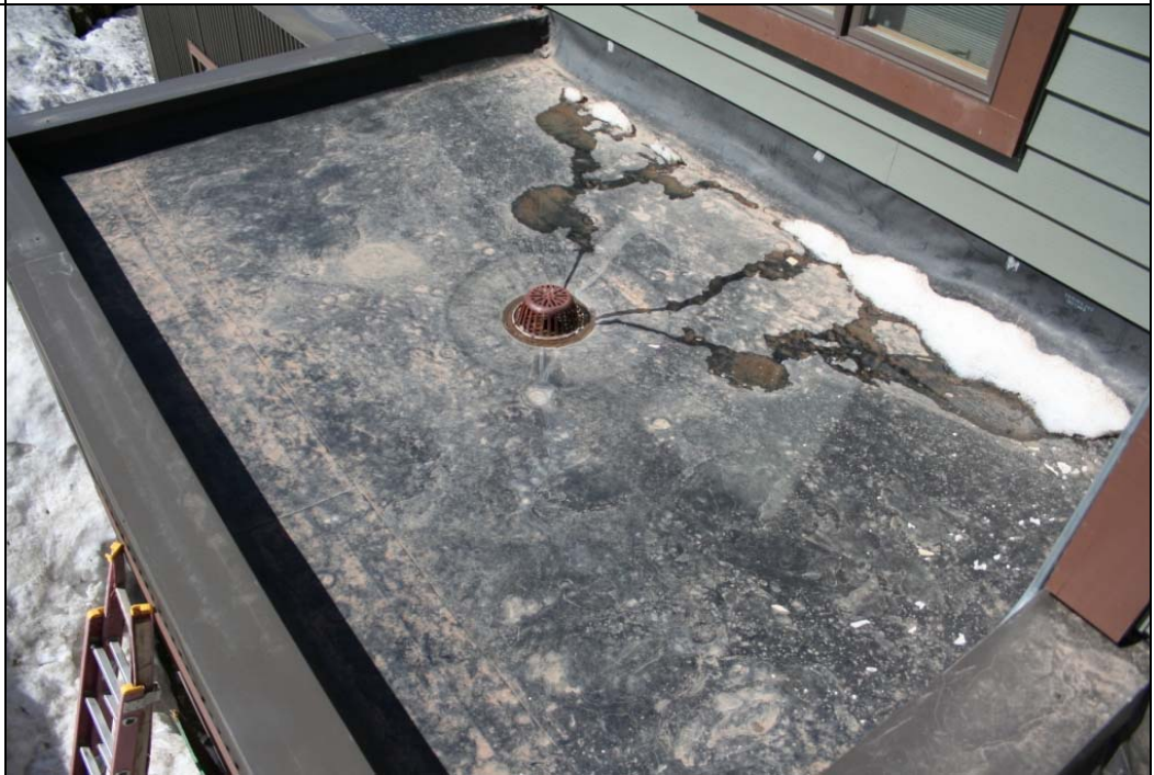
Notes: Roof Photo #1
