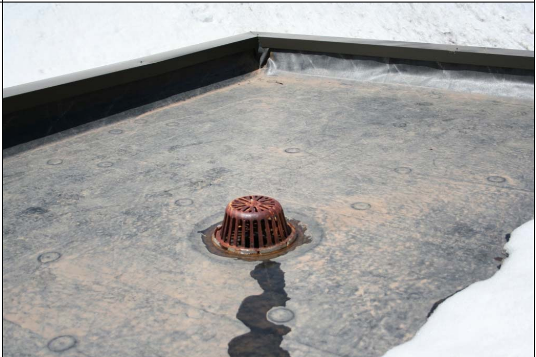
Notes: Roof Photo #2.
