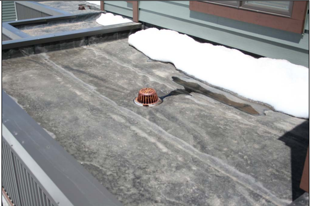
Notes: Roof Photo #1.
