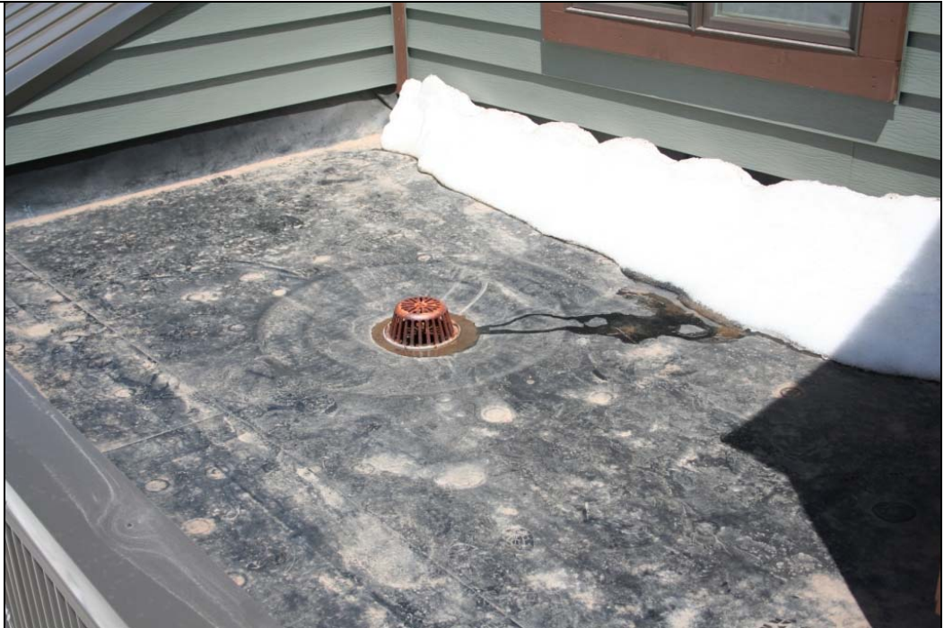
Notes: Roof Photo #2.
