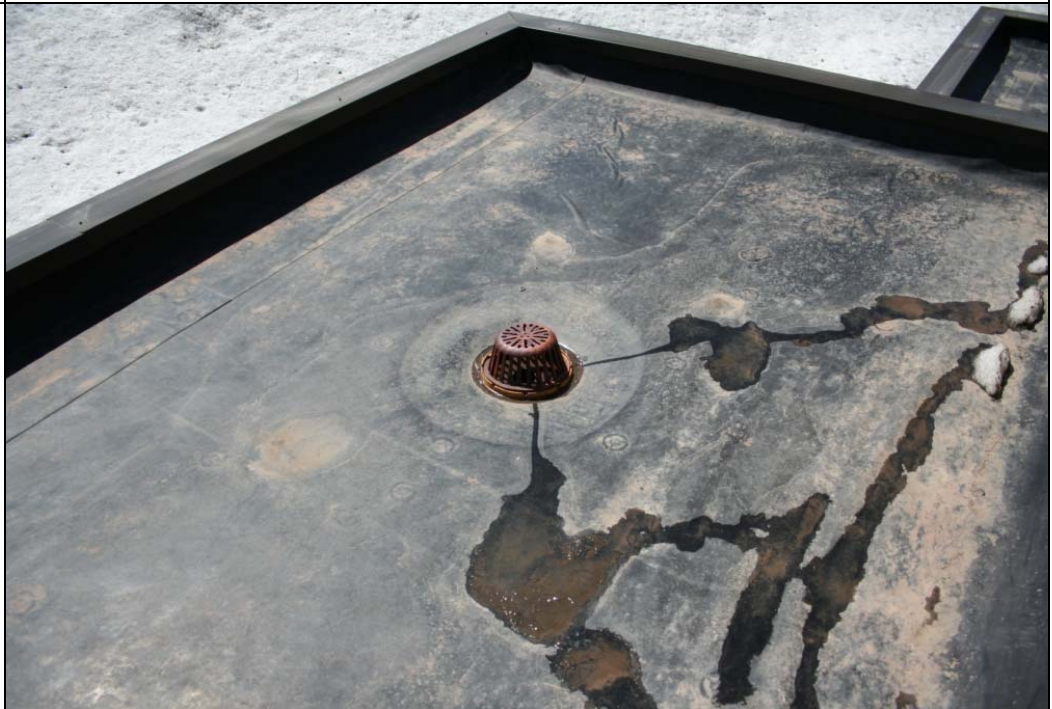
Notes: Roof Photo #2.
