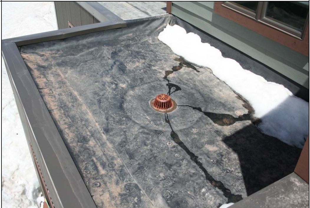
Notes: Roof Photo #1.
