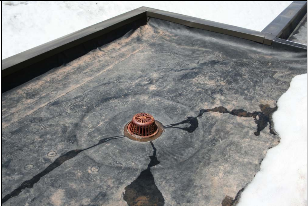
Notes: Roof Photo #2.
