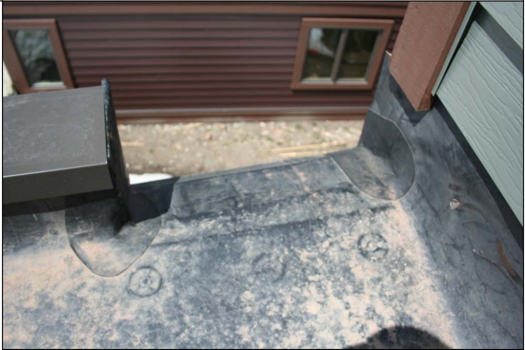
Notes: Detail of overflow scupper.
