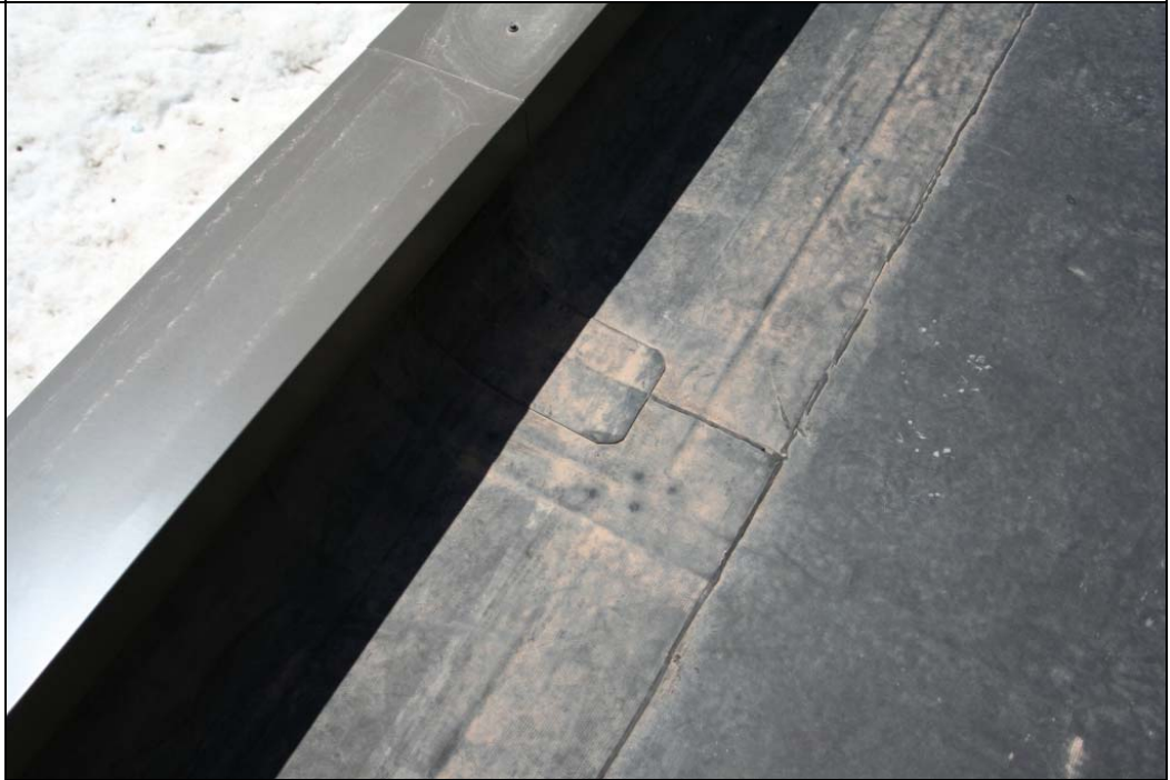
Notes: Glued seam at west centerline.
