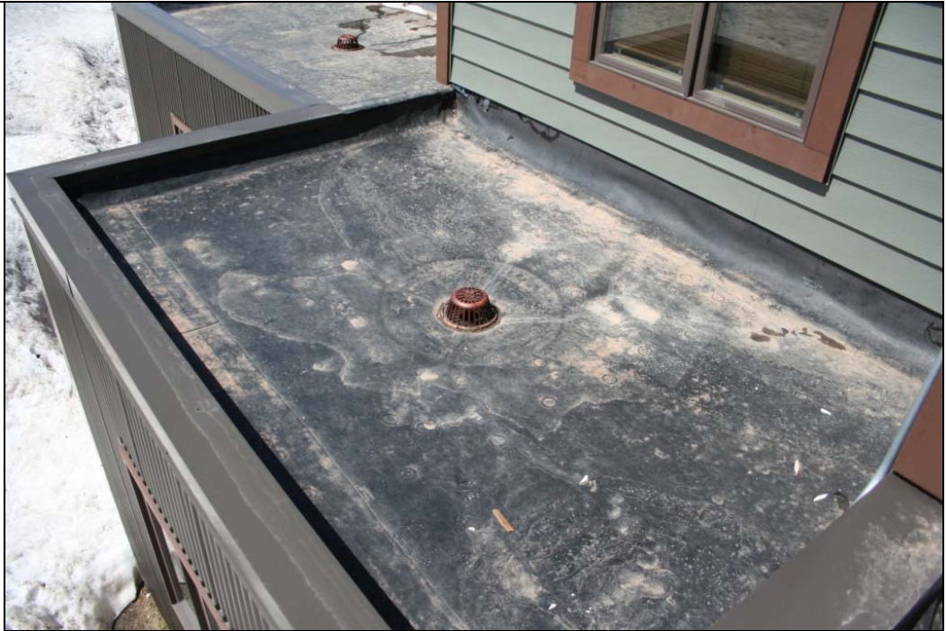
Notes: Roof Photo #1.
