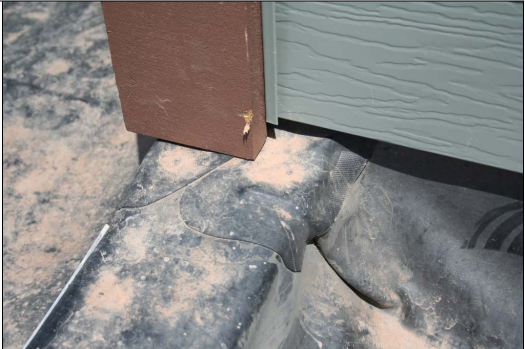
Notes: Northeast parapet cap.
