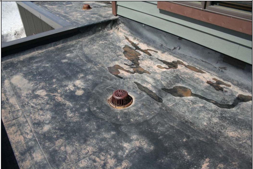
Notes: Roof Photo #2.
