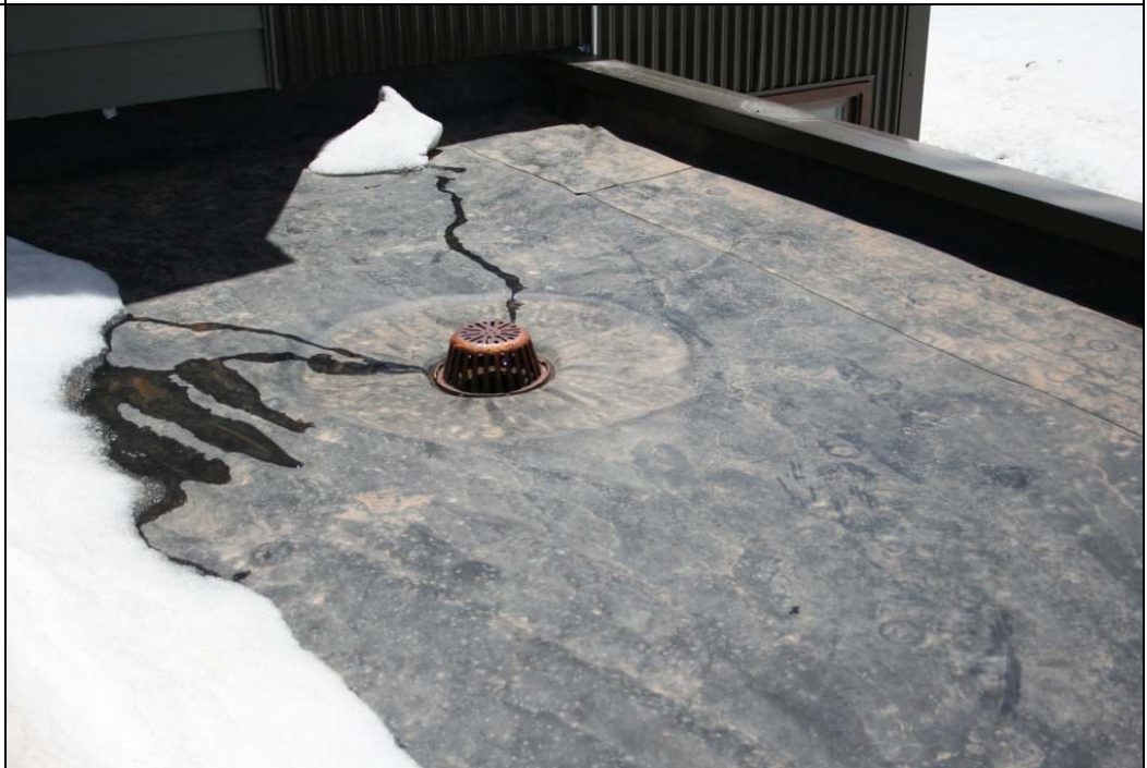
Notes: Roof Photo #2.
