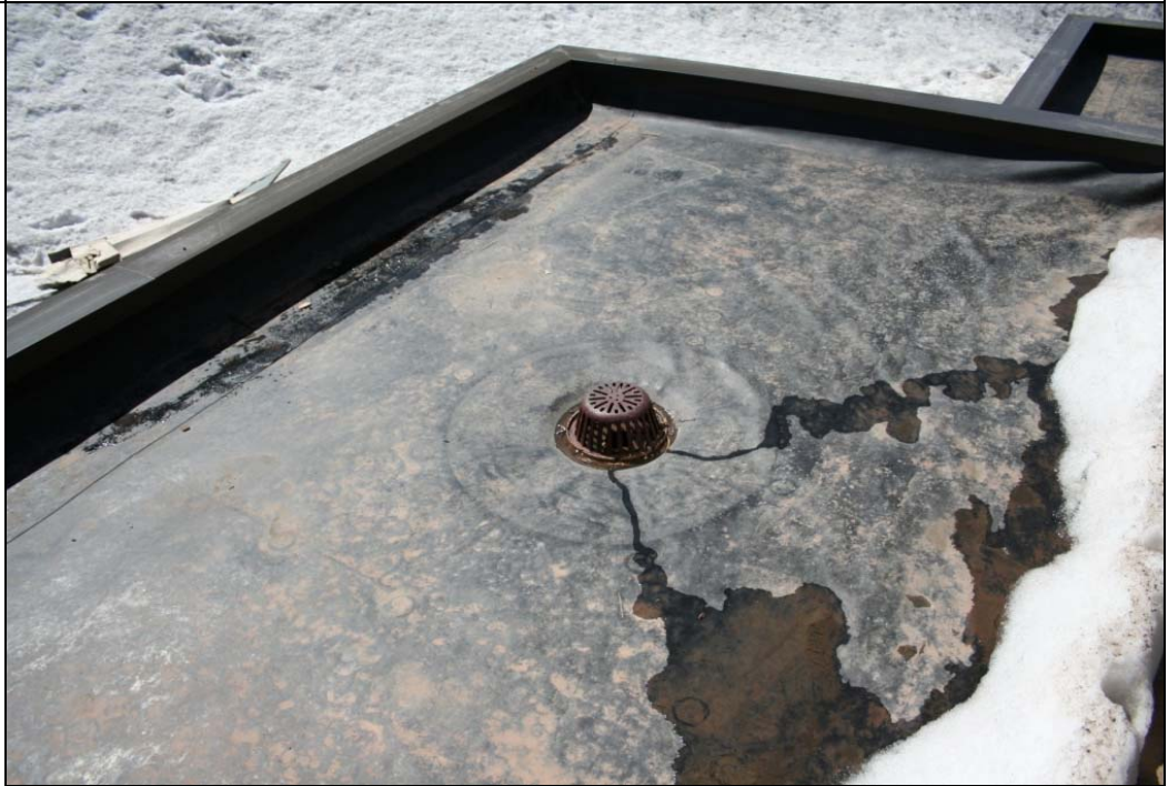
Notes: Roof Photo #2.
