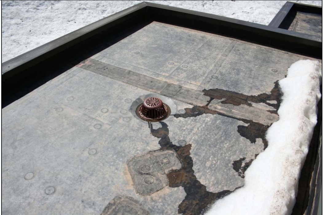
Notes: Roof Photo #2.
