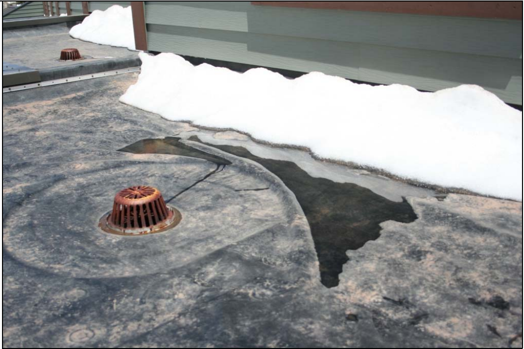
Notes: Roof Photo #1.
