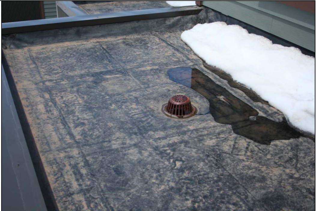
Notes: Roof Photo #1.
