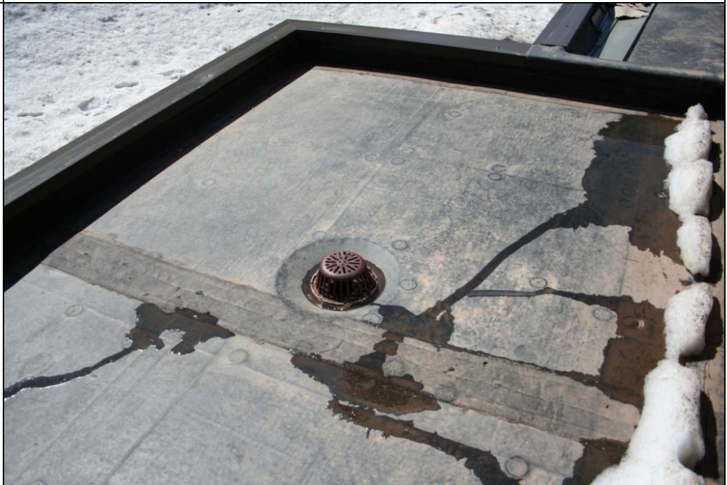
Notes: Roof Photo #2.
