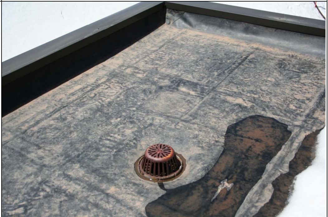
Notes: Roof Photo #2.
