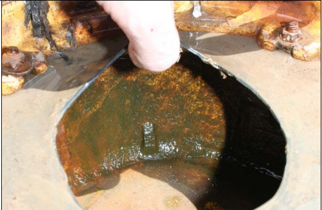
Notes: Detail of inside of roof drain.
