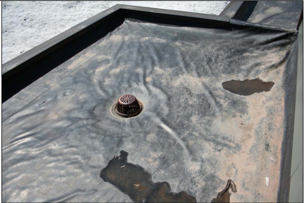
Notes: Roof Photo #2.
