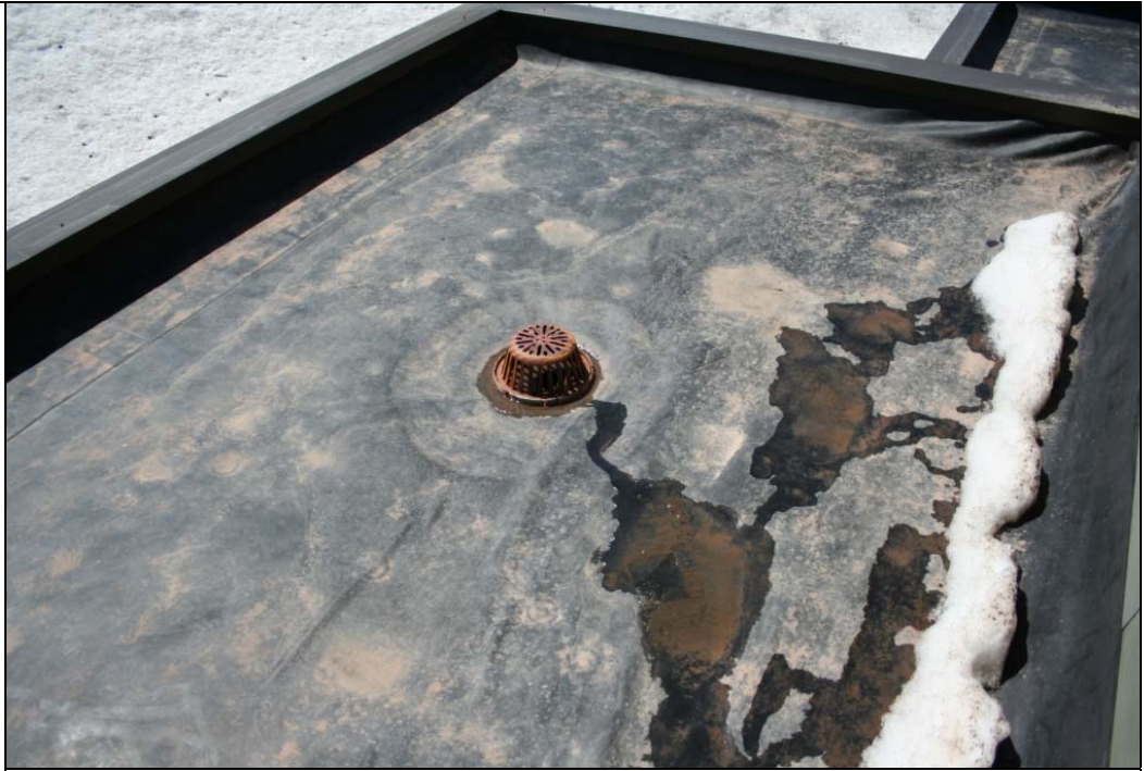
Notes: Roof Photo #2.
