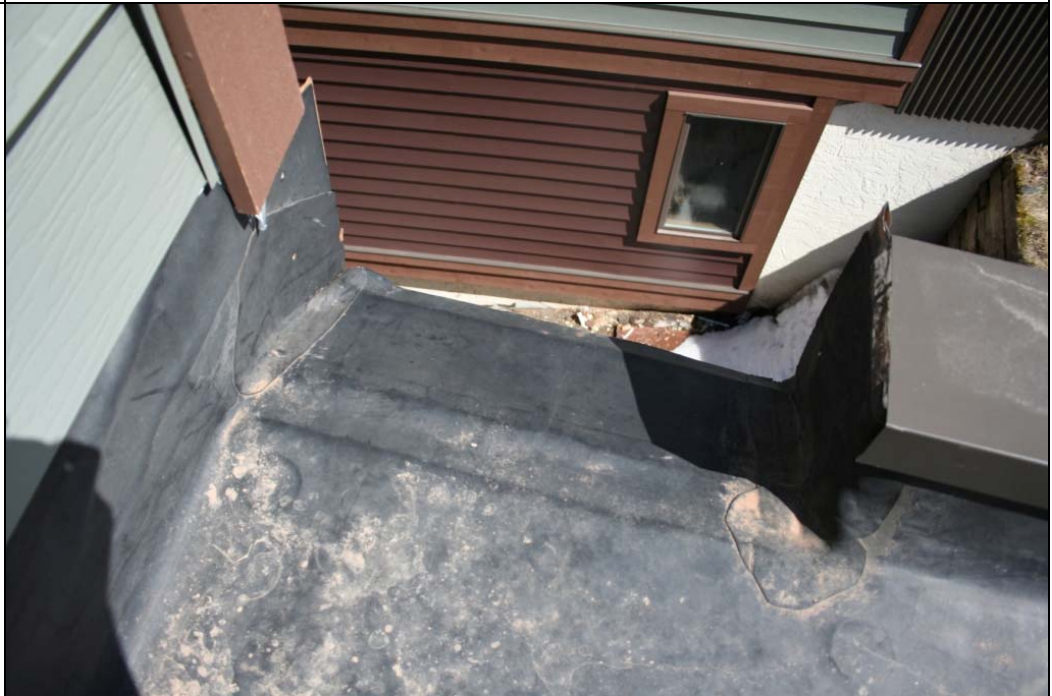
Notes: Detail of overflow scupper.
