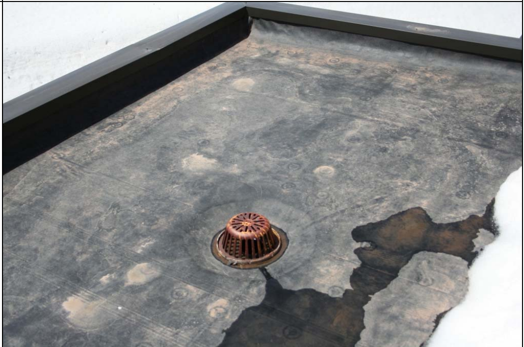
Notes: Roof Photo #2.
