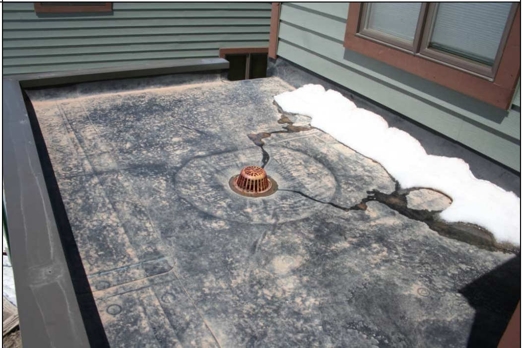
Notes: Roof Photo #1.
