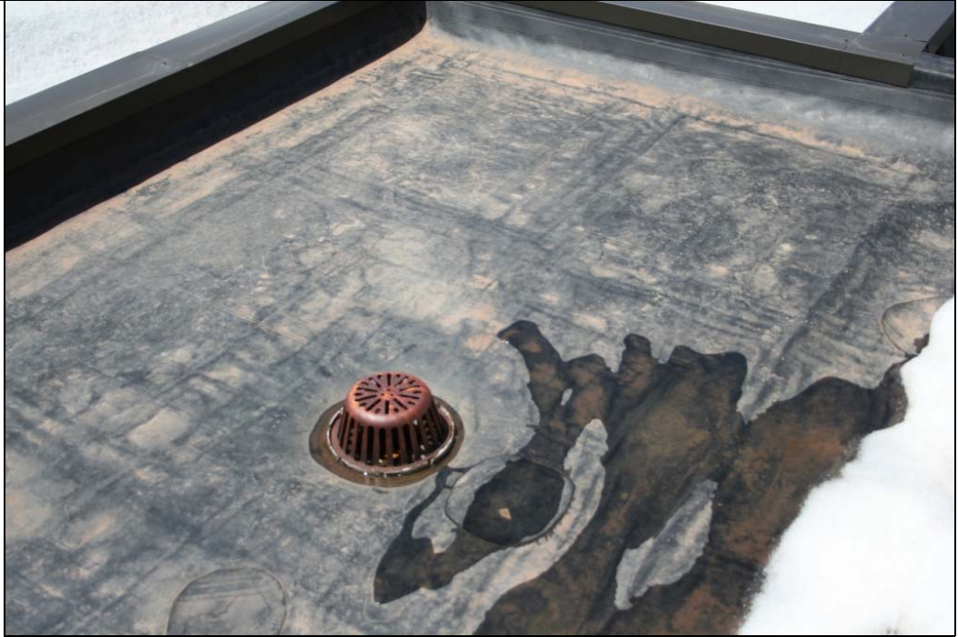
Notes: Roof Photo #1.
