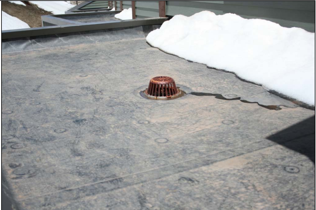
Notes: Roof Photo #1.
