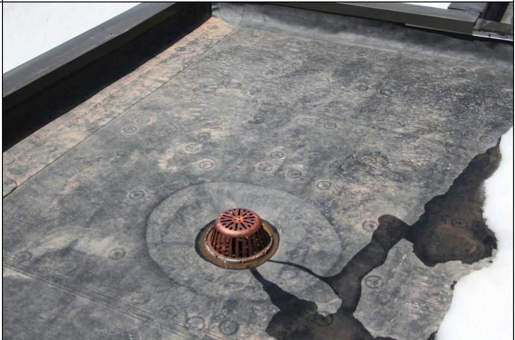
Notes: Roof Photo #2.
