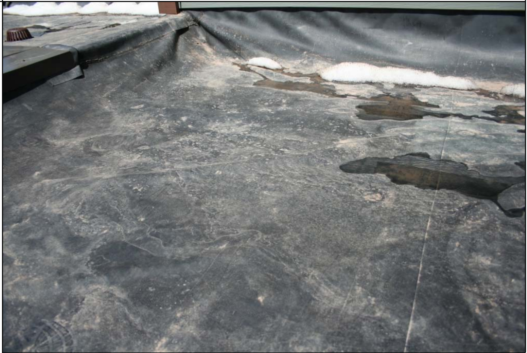
Notes: Membrane is not adhered to substrate.
