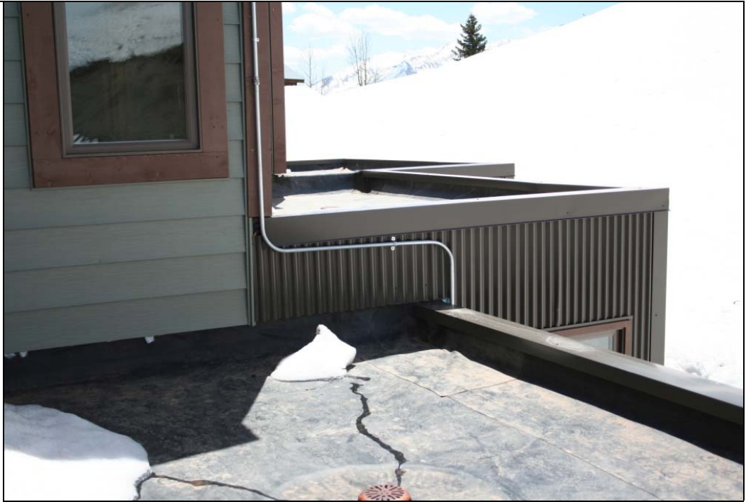
Notes: Roof Photo #3.
