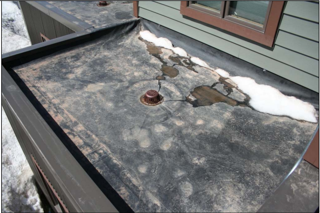
Notes: Roof Photo #1.
