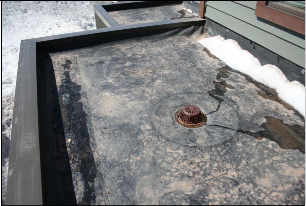
Notes: Roof Photo #1.
