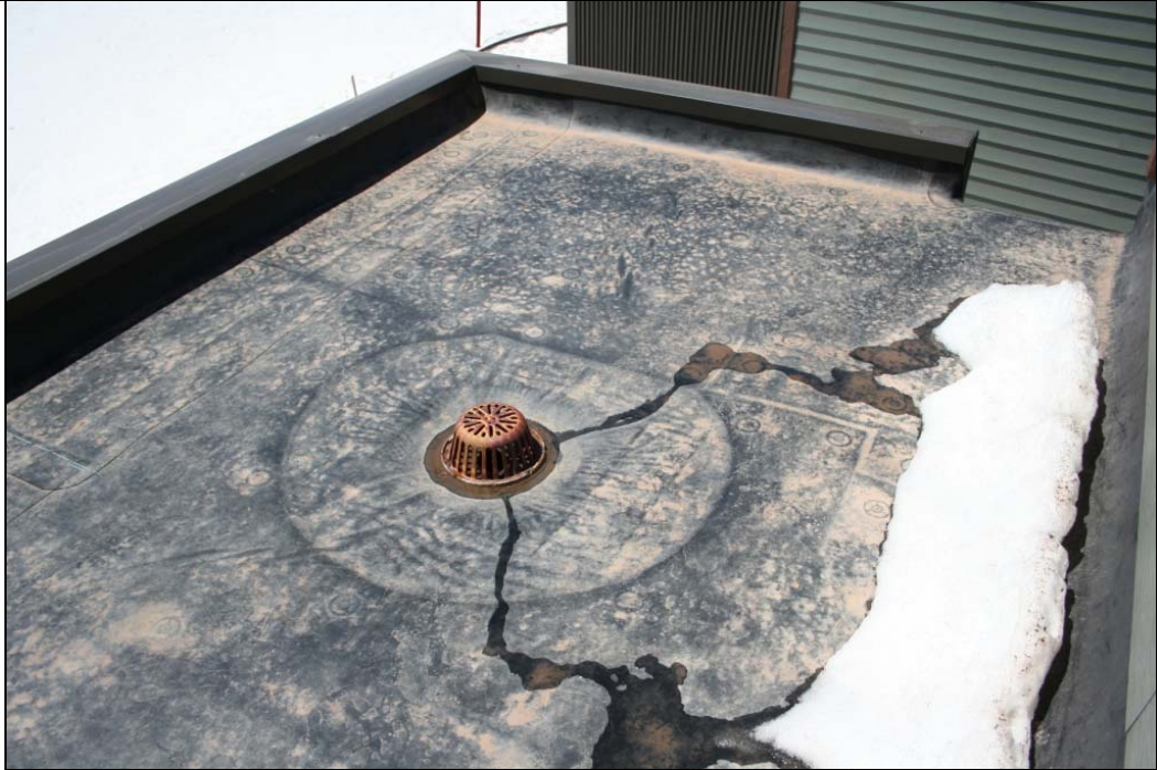
Notes: Roof Photo #2.
