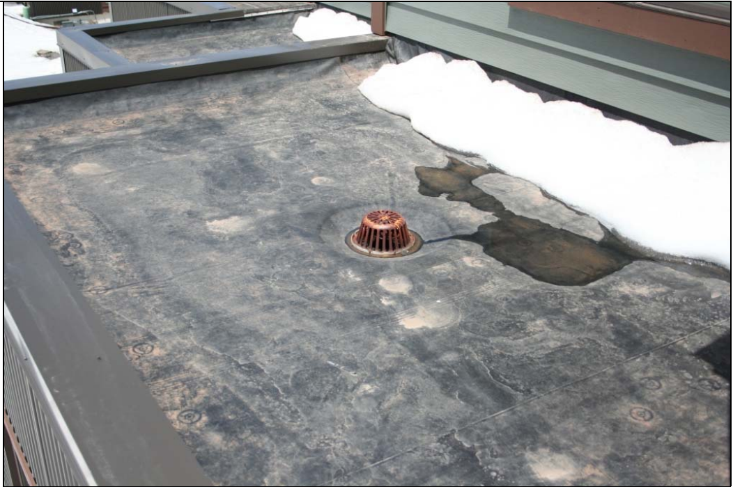
Notes: Roof Photo #1.
