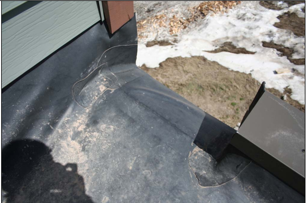
Notes: Overflow scupper detail.
