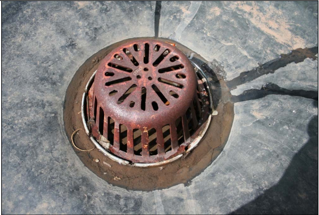
Notes: Roof drain detail.
