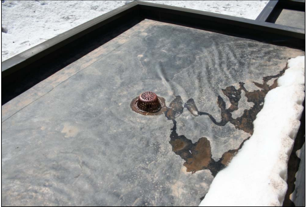
Notes: Roof Photo #2.
