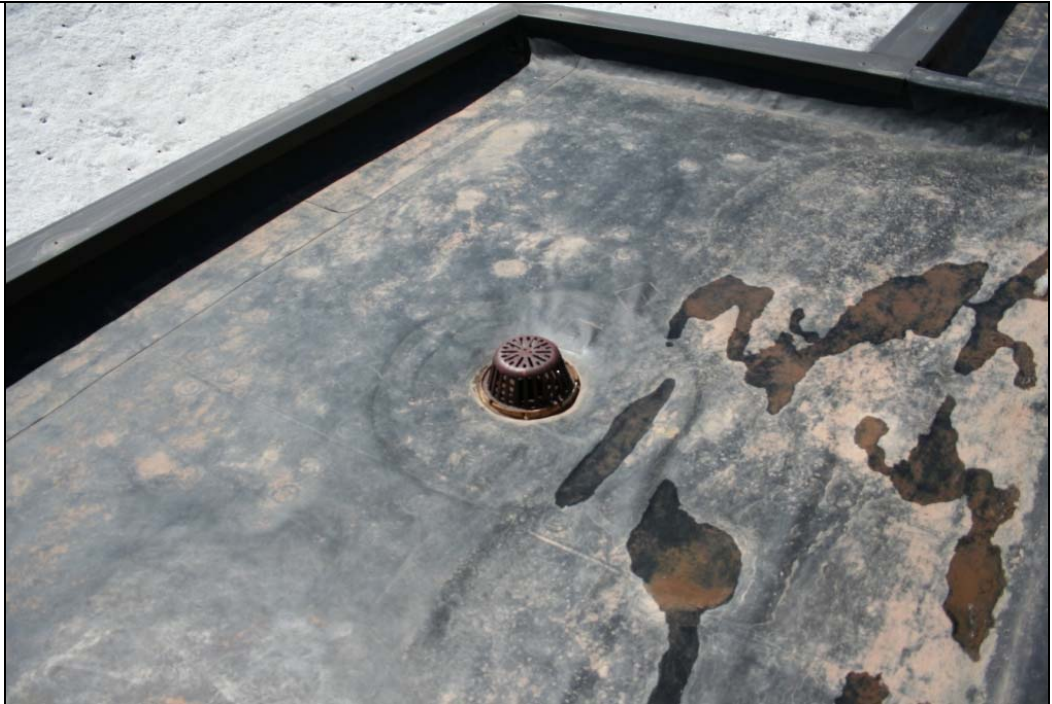
Notes: Roof Photo #1.
