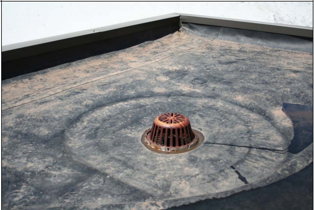
Notes: Roof Photo #2.
