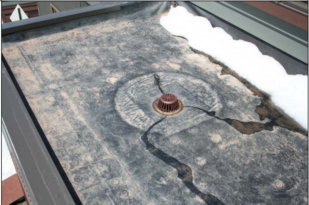
Notes: Roof Photo #1.
