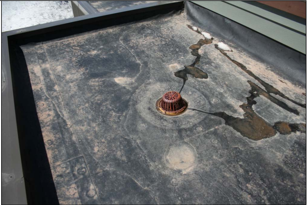
Notes: Roof Photo #1.
