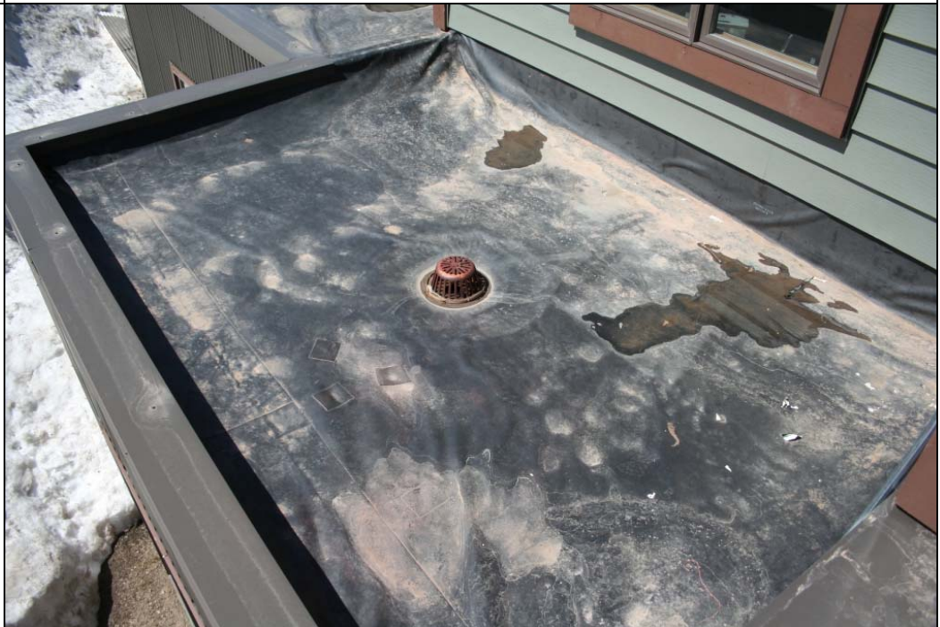
Notes: Roof Photo #1.
