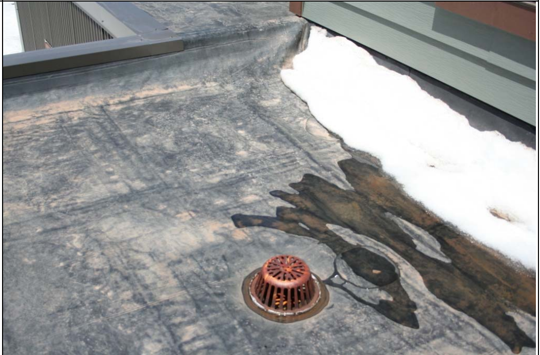
Notes: Roof Photo #2.
