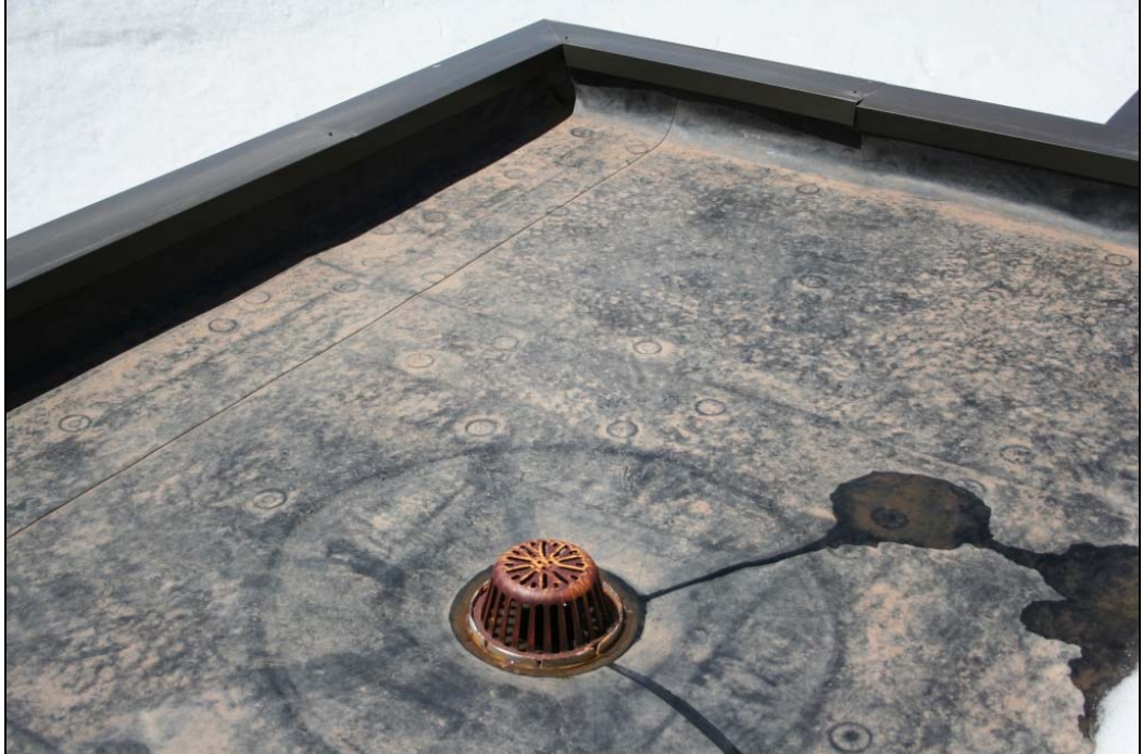
Notes: Roof Photo #2.
