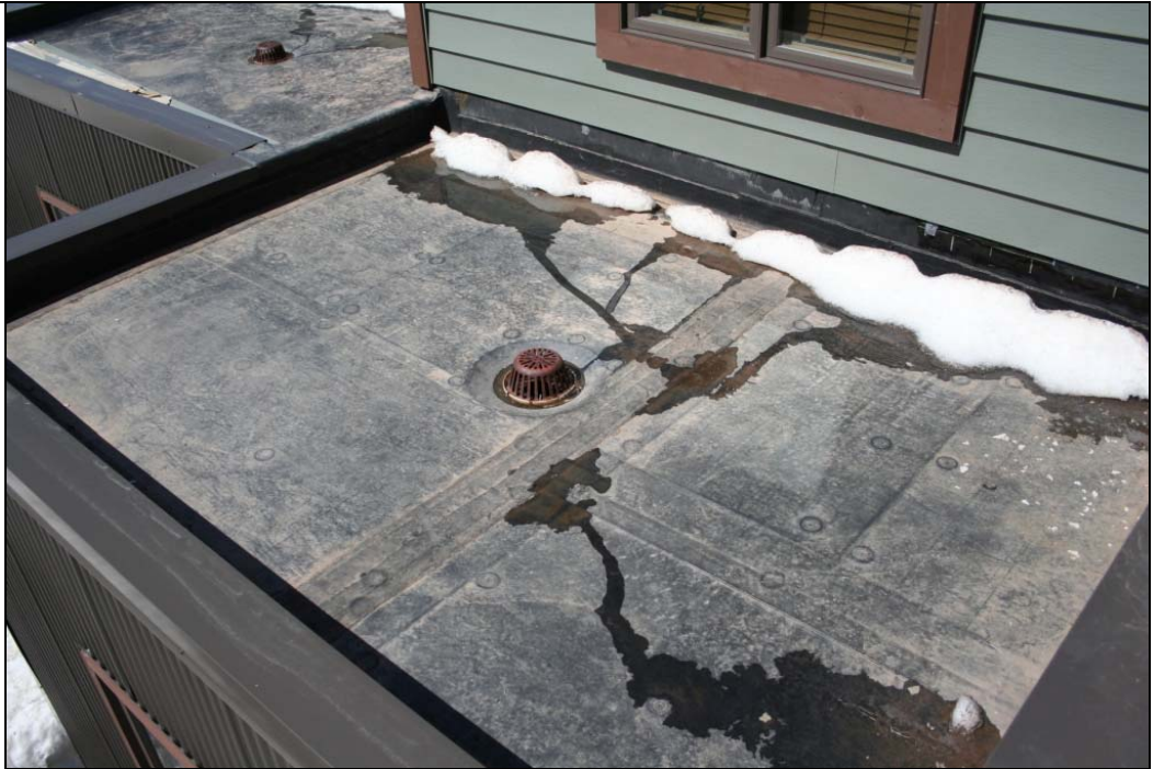
Notes: Roof Photo #1.
