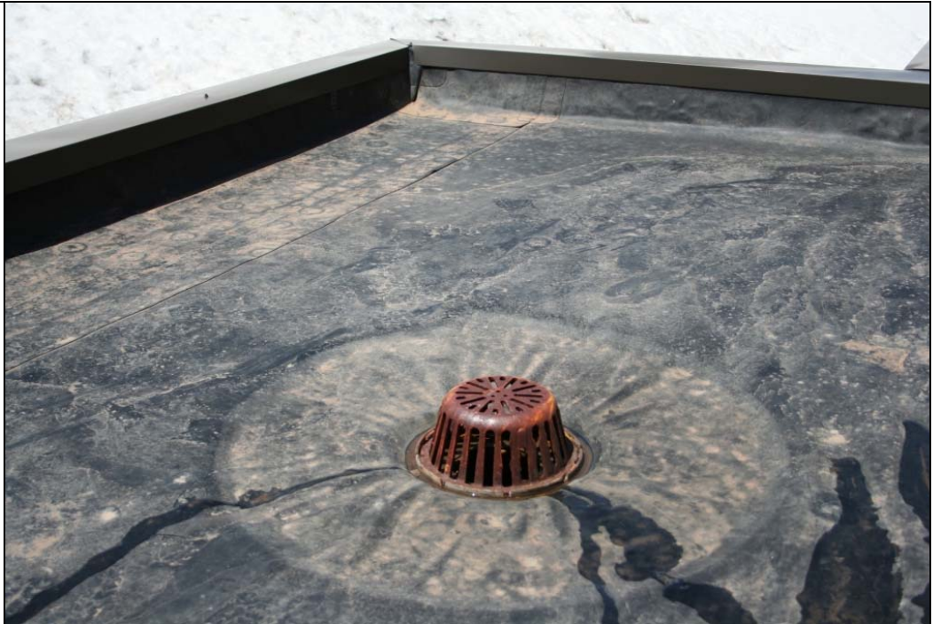
Notes: Roof Photo #1.
