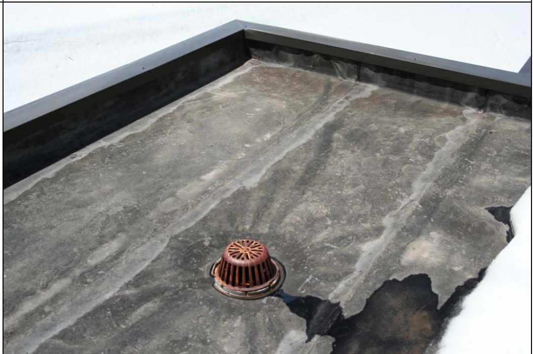
Notes: Roof Photo #2.
