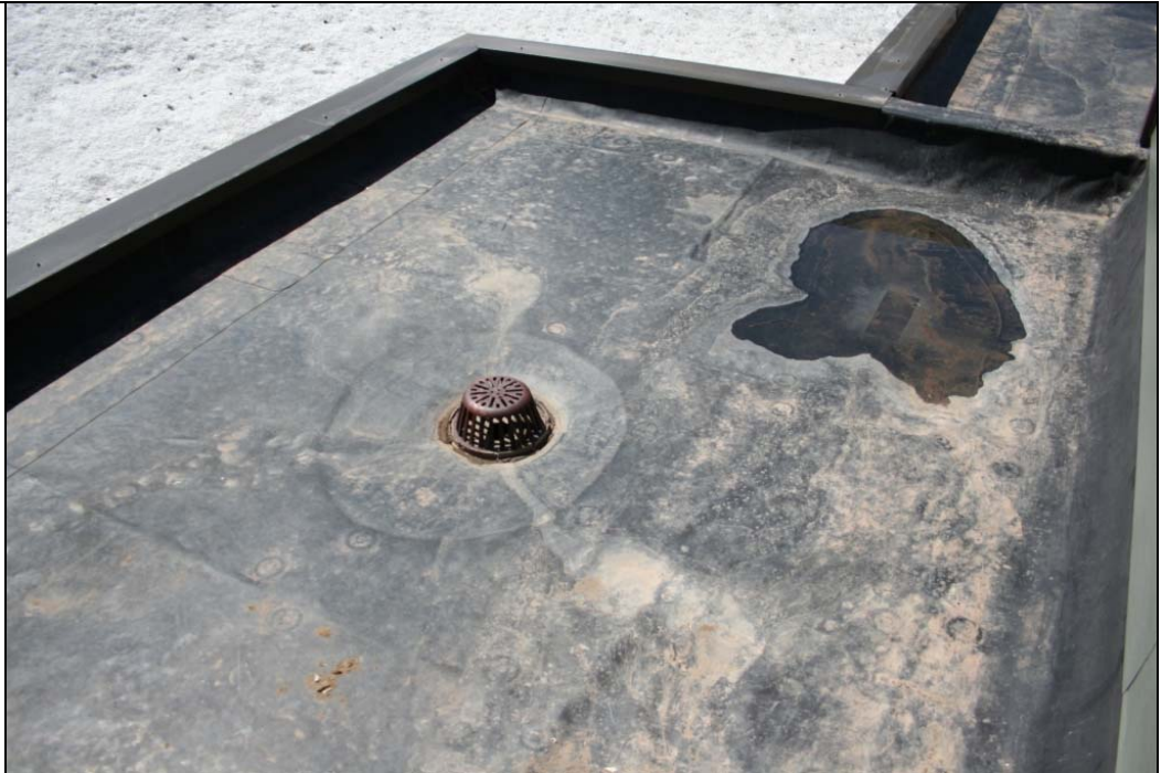
Notes: Roof Photo #2.
