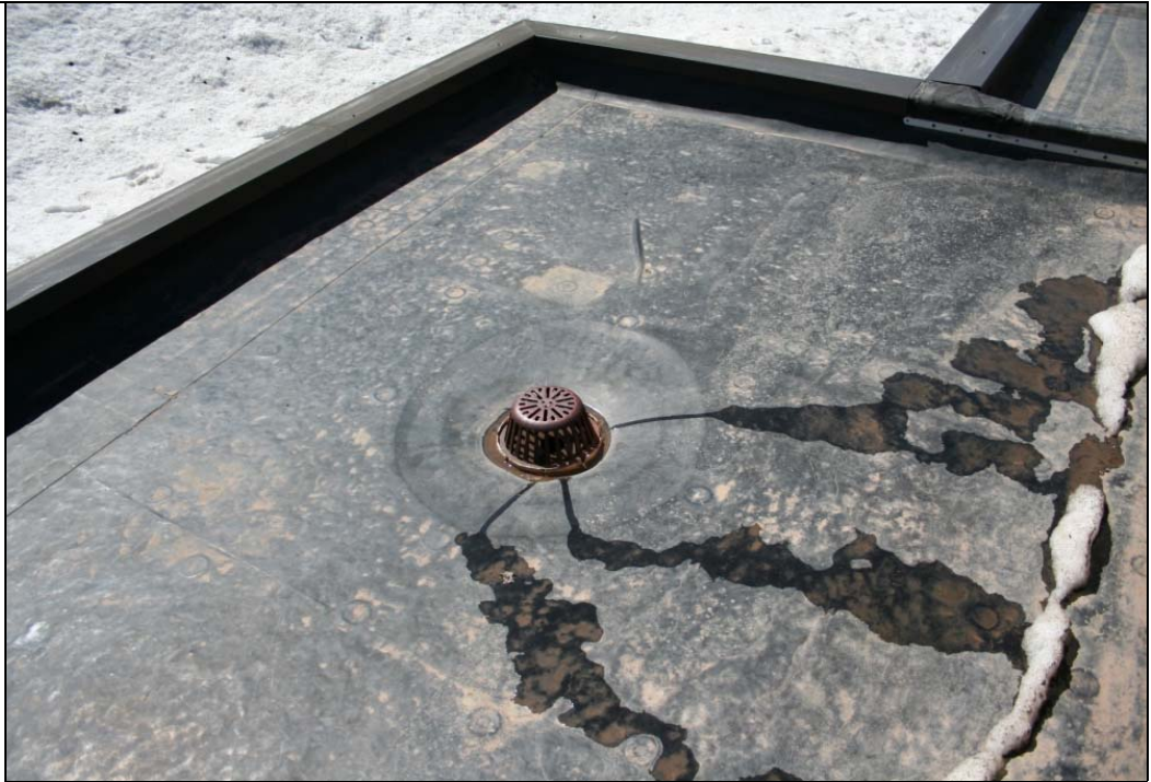
Notes: Roof Photo #2.
