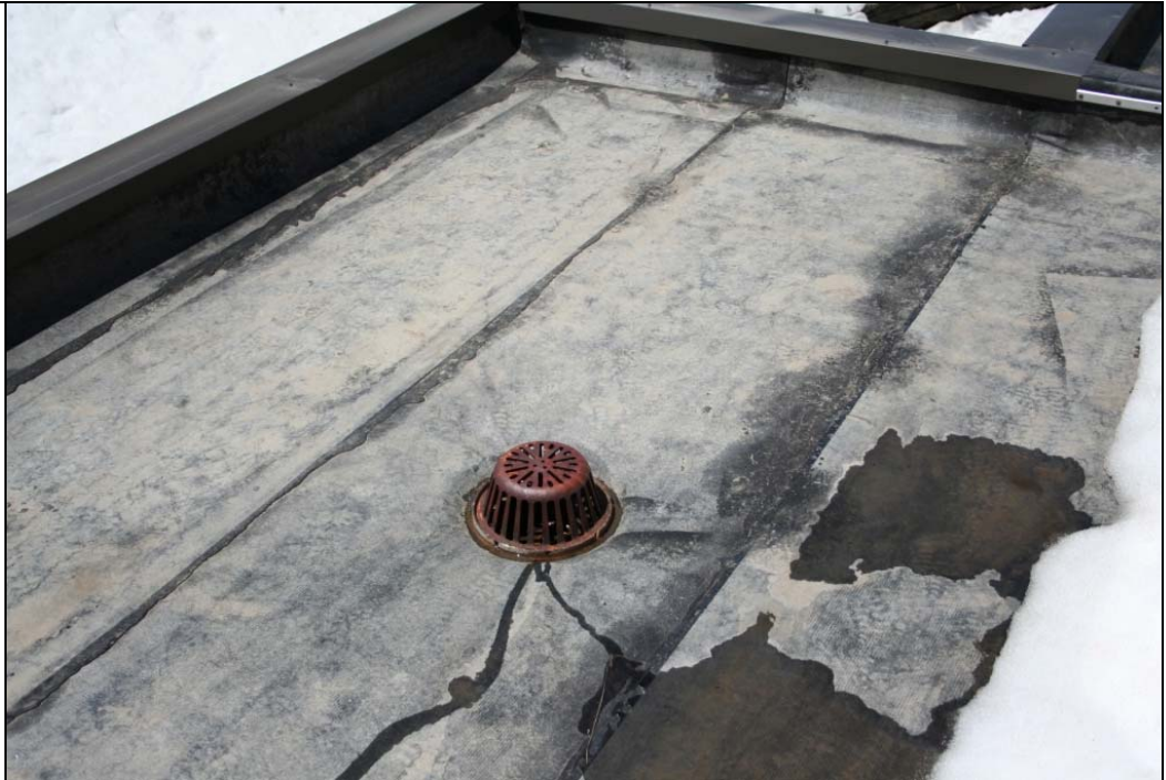
Notes: Roof Photo #2.
