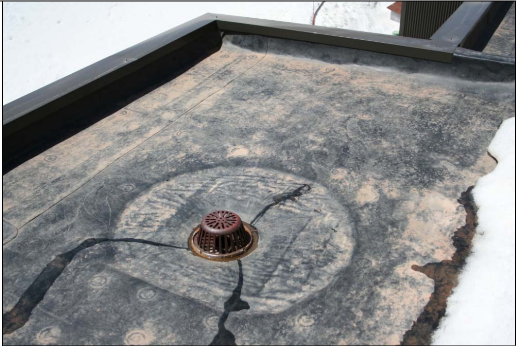
Notes: Roof Photo #2.
