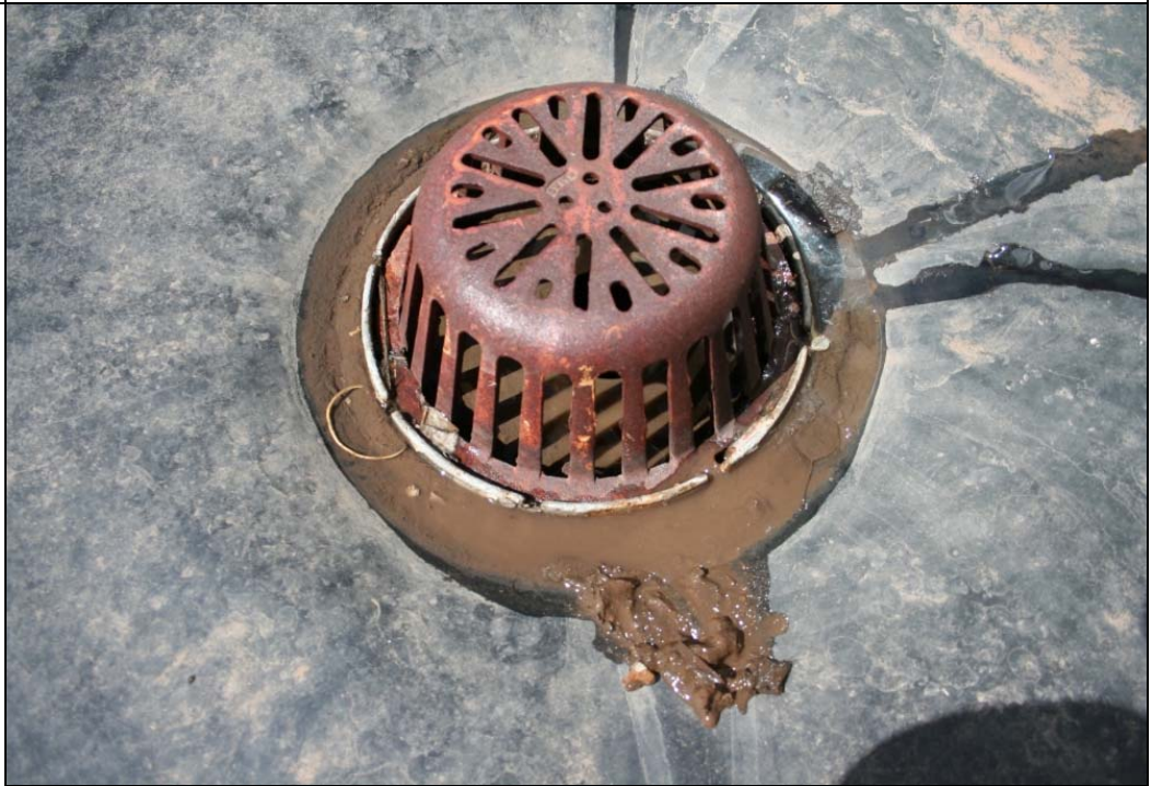
Notes: Debris and dirt removed from outside ring of roof drain.
