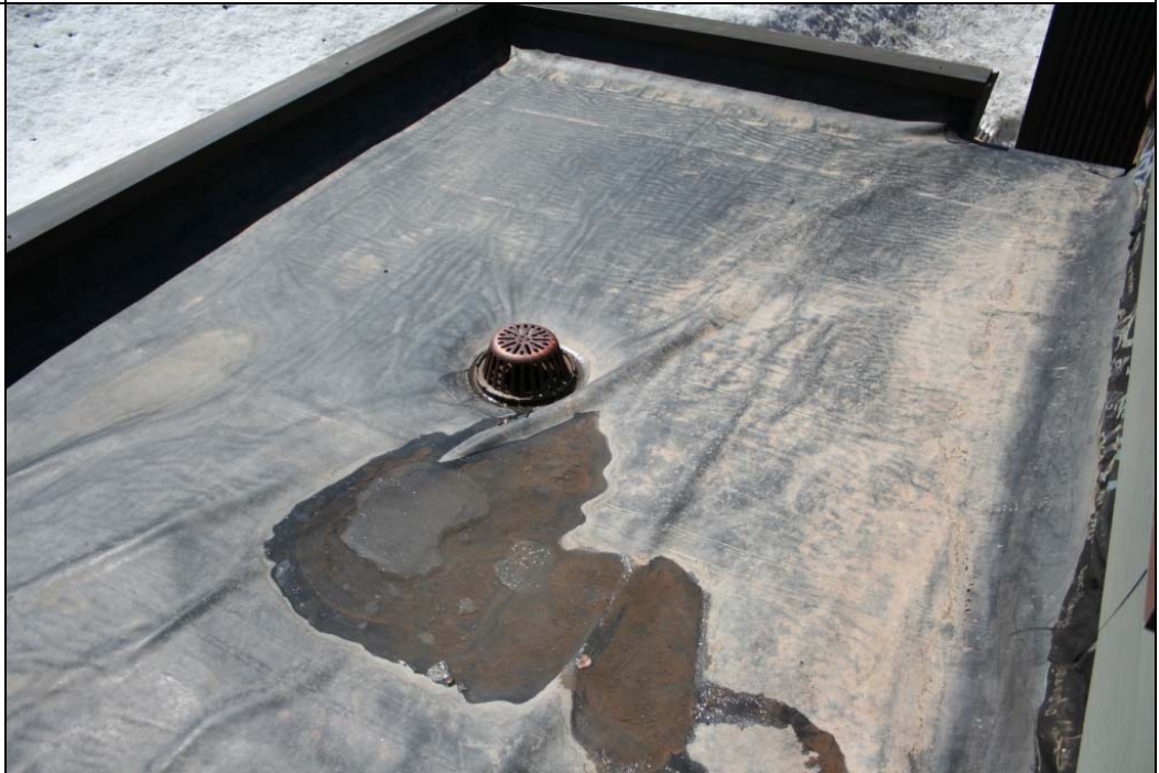
Notes: Roof Photo #2
