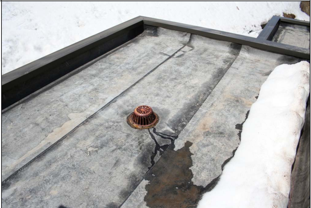
Notes: Roof Photo #2.
