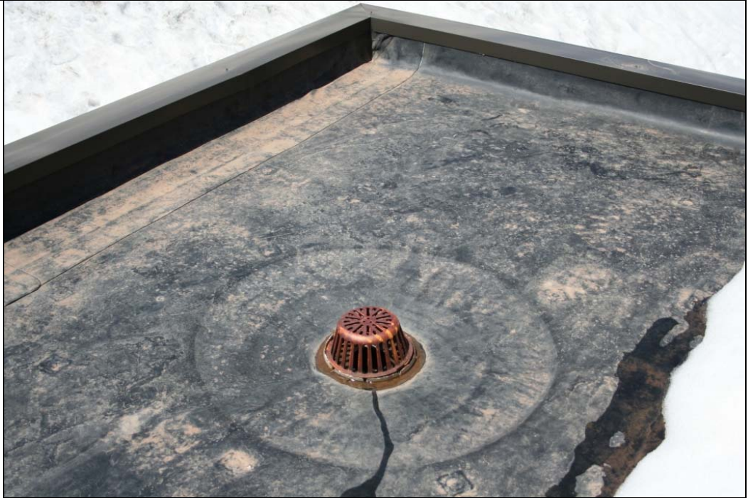
Notes: Roof Photo #2.
