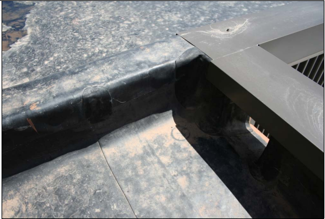
Notes: Patch at seam on south parapet wall near overflow scupper.
