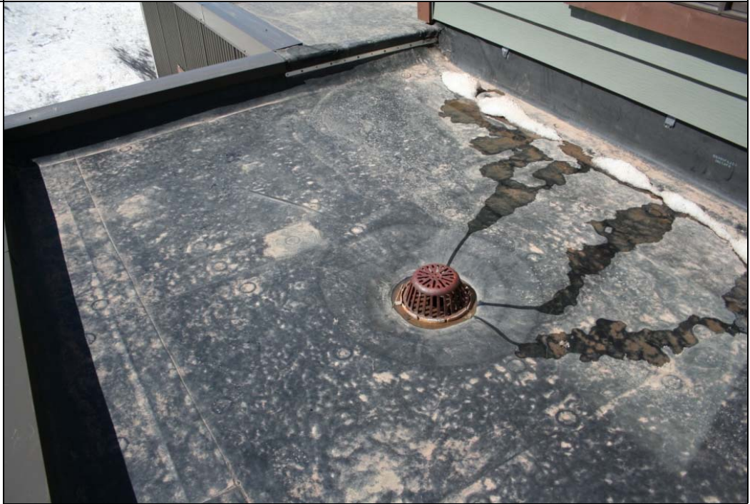
Notes: Roof Photo #1.
