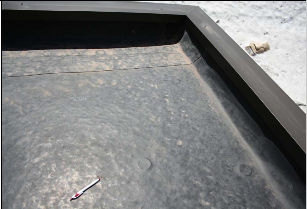
Notes: Hole 3-'6" north of drain.
