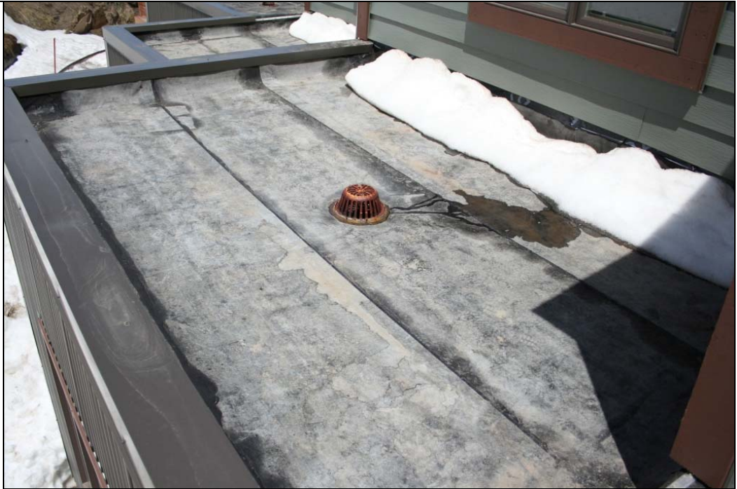
Notes: Roof Photo #1.
