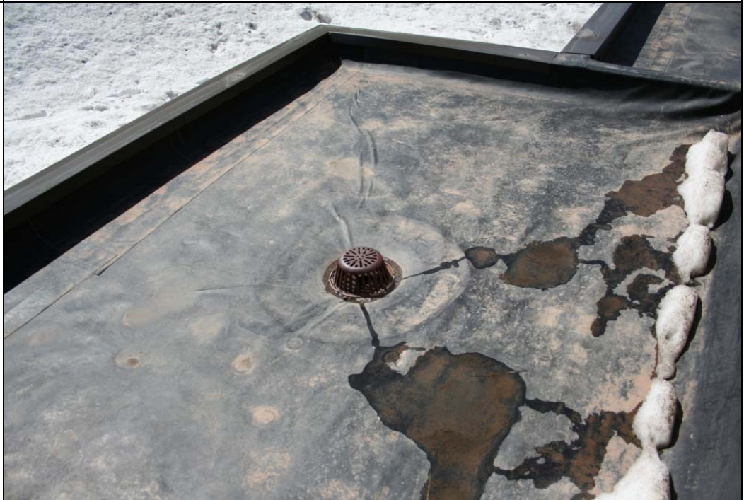
Notes: Roof Photo #2.
