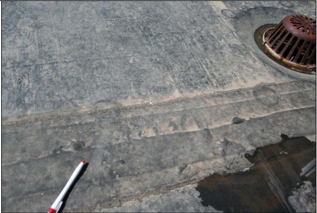
Notes: Bubbling in seam. Multiple locations.
