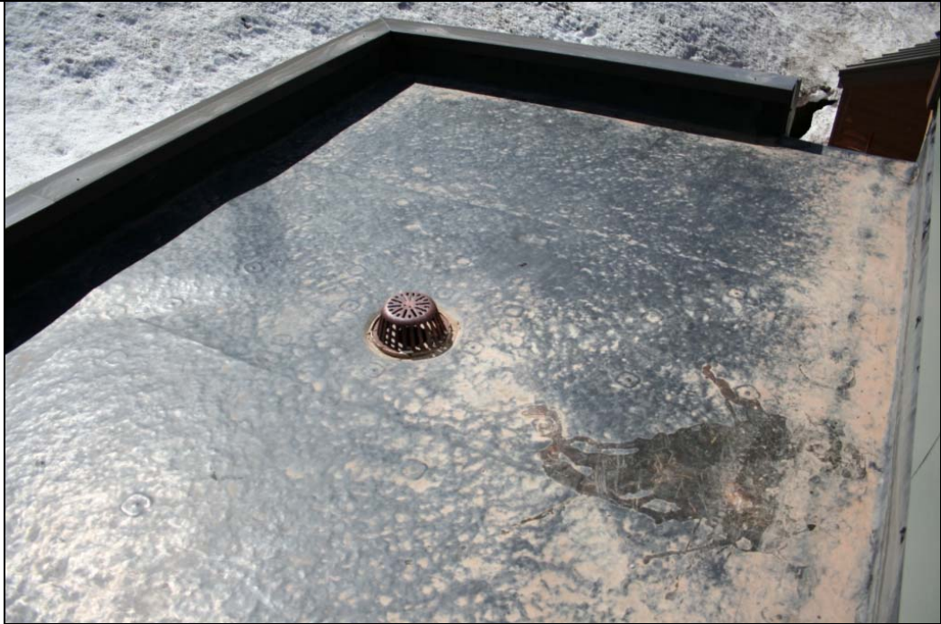
Notes: Roof Photo 2
