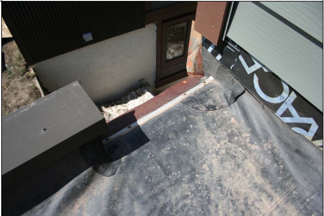
Notes: Detail of overflow scupper.
