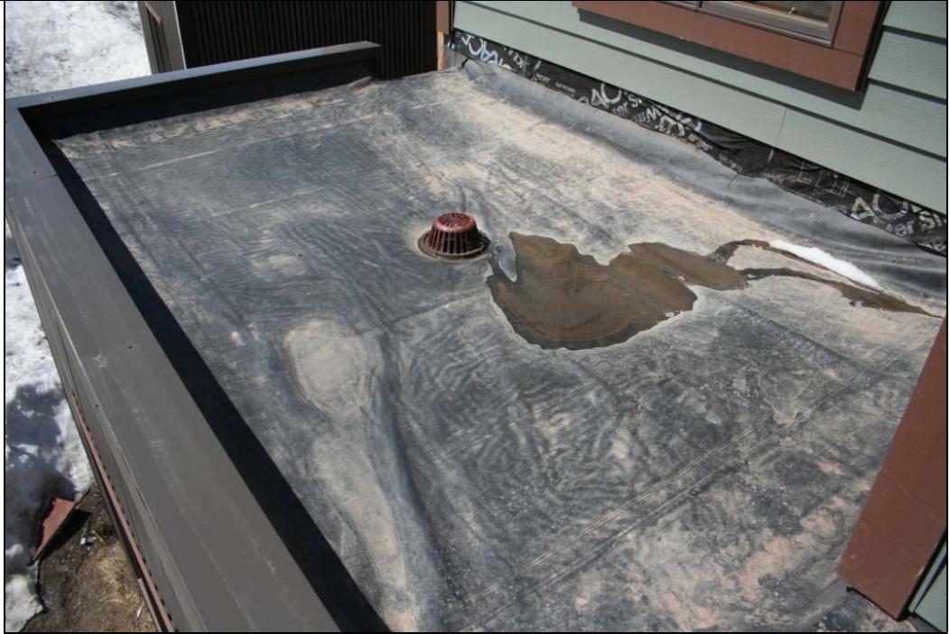
Notes: Roof Photo #1
