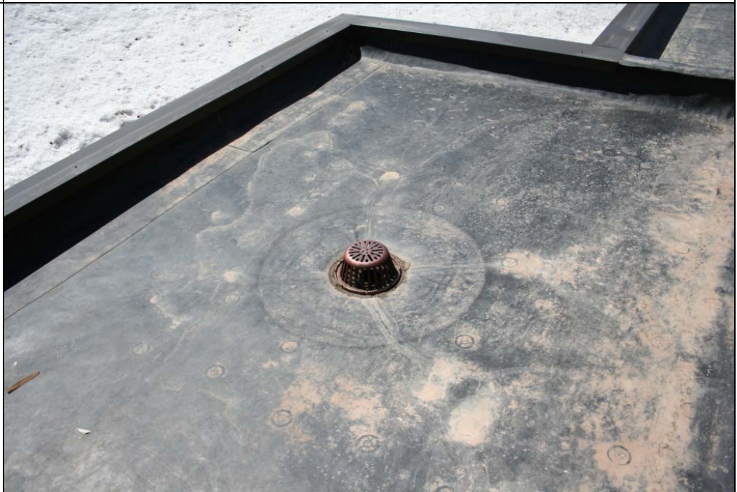
Notes: Roof Photo #2.
