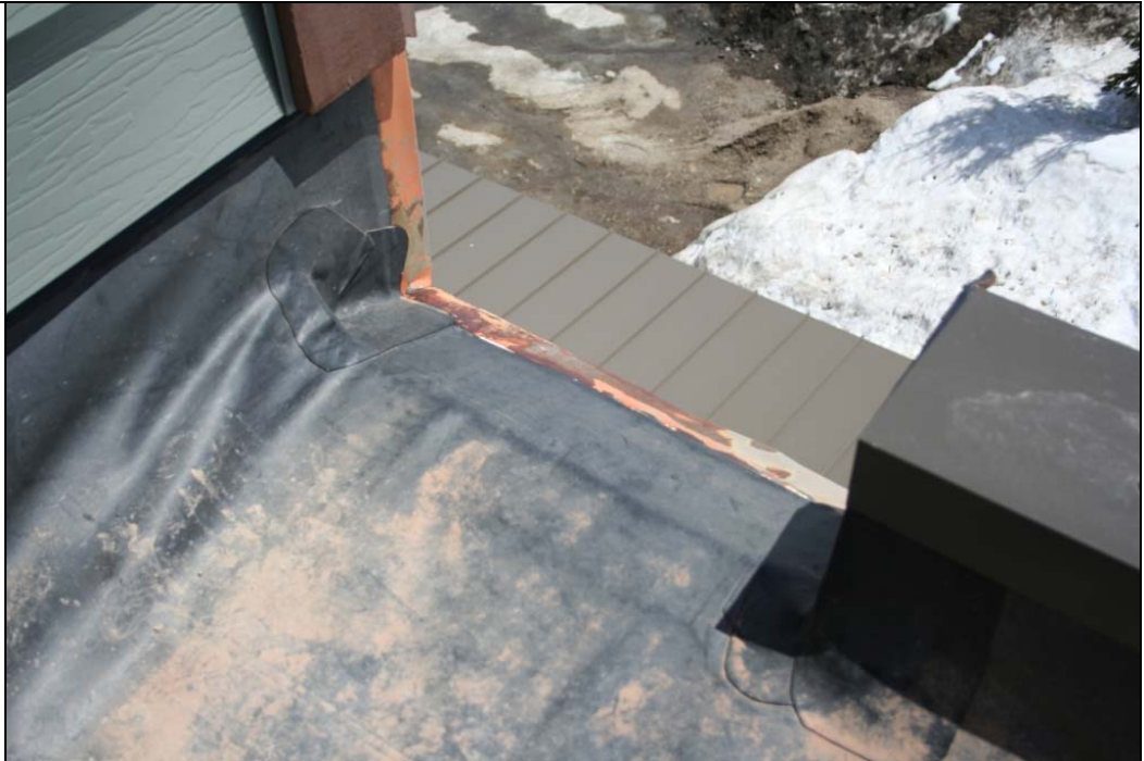
Notes: Detail of overflow scupper on south parapet wall.
