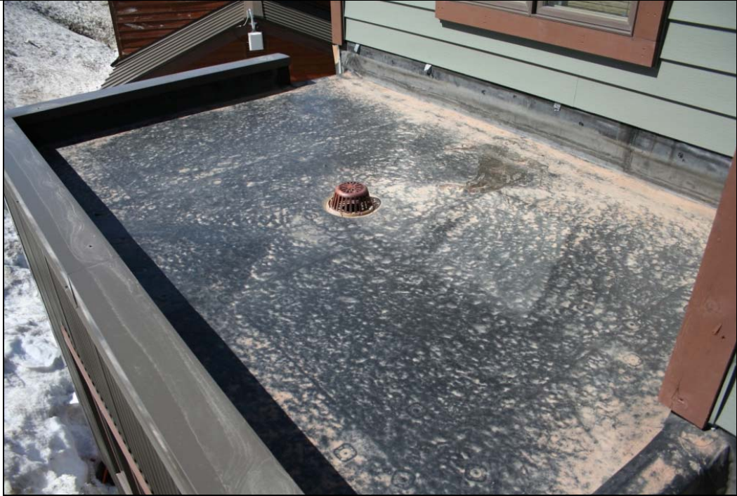
Notes: Roof Photo 1
