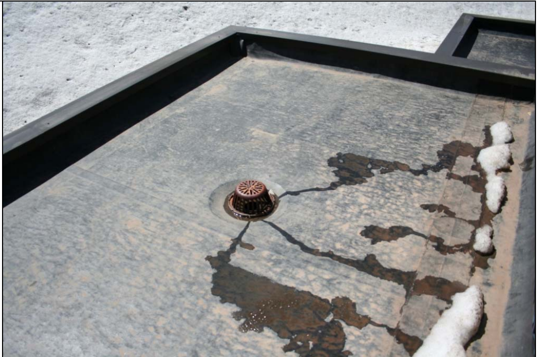
Notes: Roof Photo #2.
