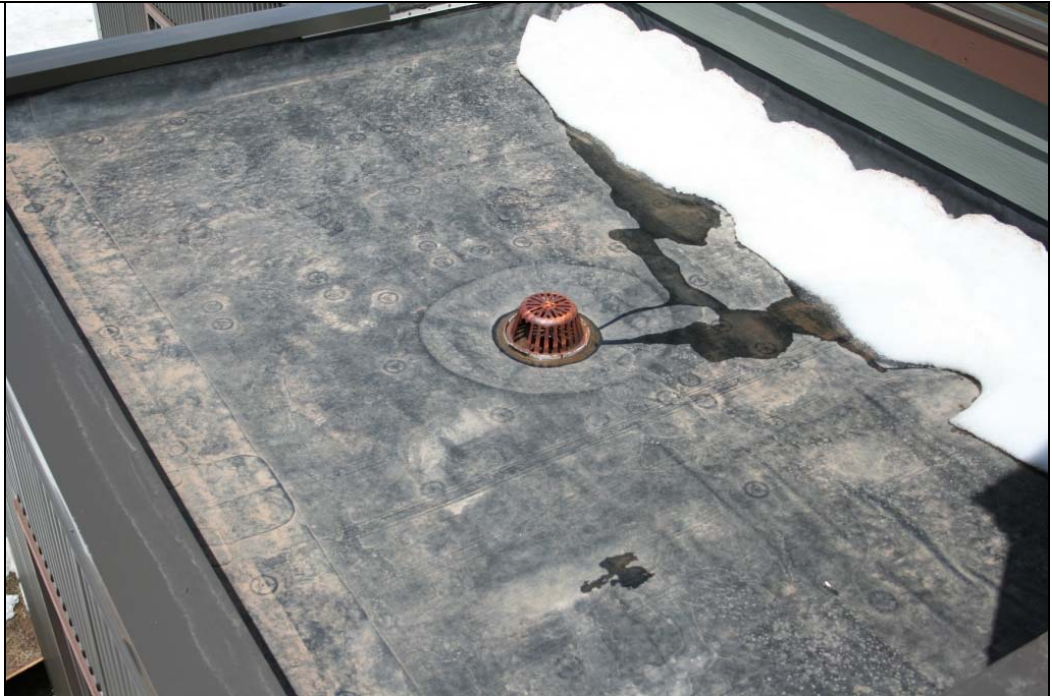
Notes: Roof Photo #1.
